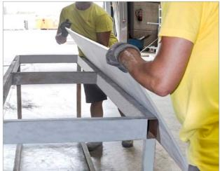
Image 9: Placing a Neolith Slab on a bench
